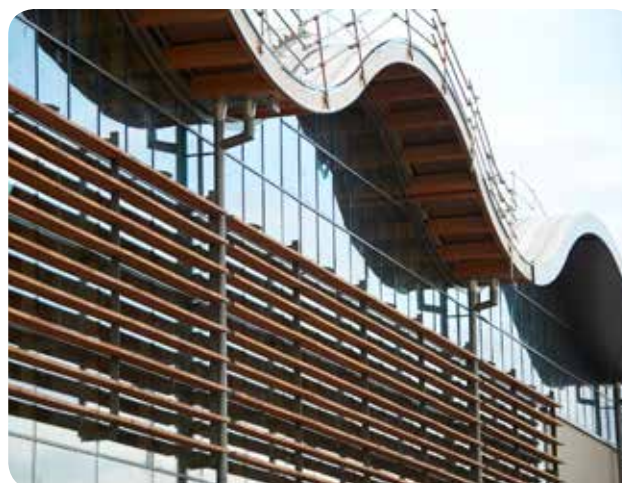
Figure 1: The Marks and Spencer store at Cheshire Oaks, near Ellesmere Port, constructed by Simons Group. Only FSC certified wood was used (FSC project licence: TT-PRO-003615:2012)
