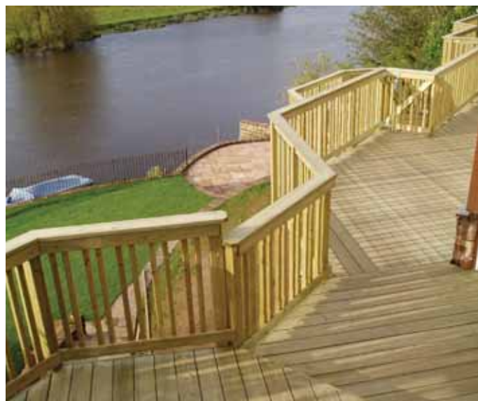
A multi-level waterside deck. Photo: Timber Decking and Cladding Association
