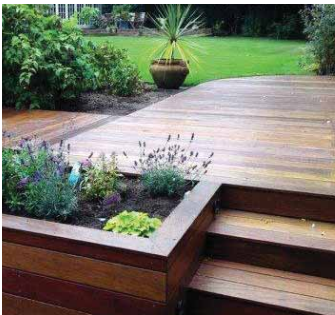
Ipe hardwood decking provides a contemporary feel to the garden. Ipe is categorised with Class 1 natural durability. Photo: Silva Timber
